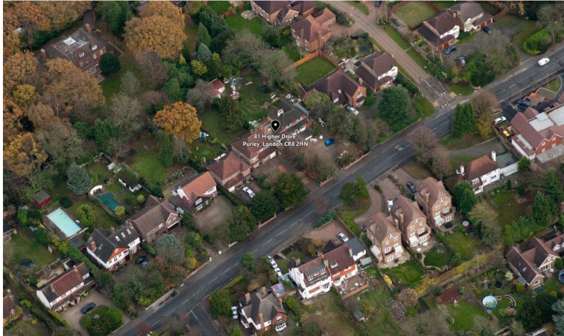
Fig 1: Aerial street view highlighting the proposed site within the surrounding streetscene
